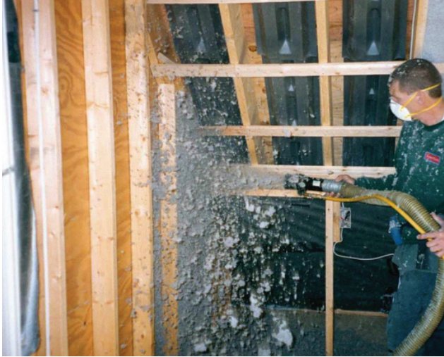
Roof line venting chute.
