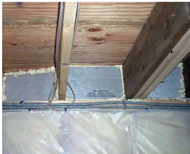
Rim joist sealed to sill.
