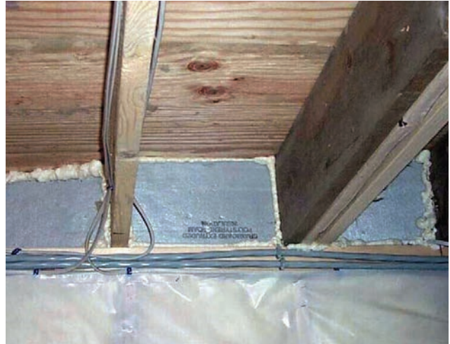
Rim joist insulated (and sealed to sill) with foam board and one-part foam.
