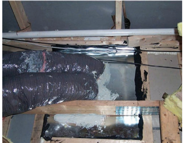
Open attic chase sealed with sheet metal, duct mastic, and acoustical sealant.
