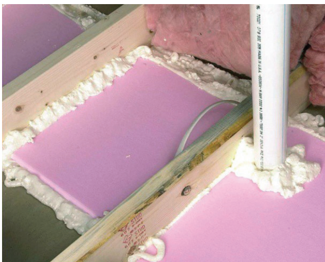
Dropped soffit sealed with extruded polystyrene insulation (XPS) and one-part foam.
