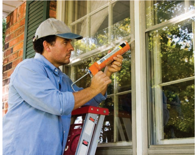
Applying caulk around window frame.
