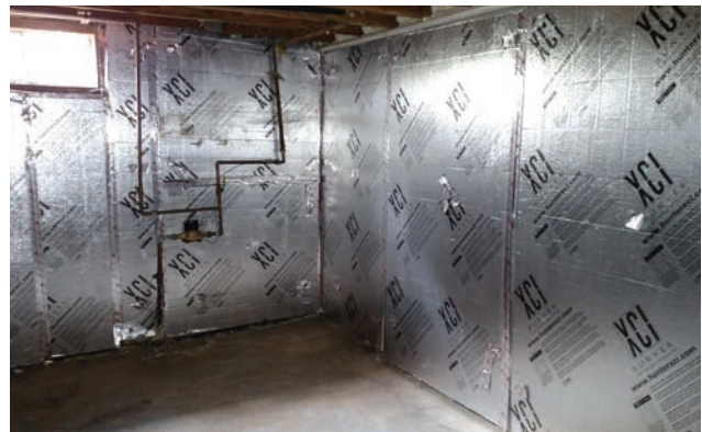
Basement and crawlspace insulation interior wall treatment.
