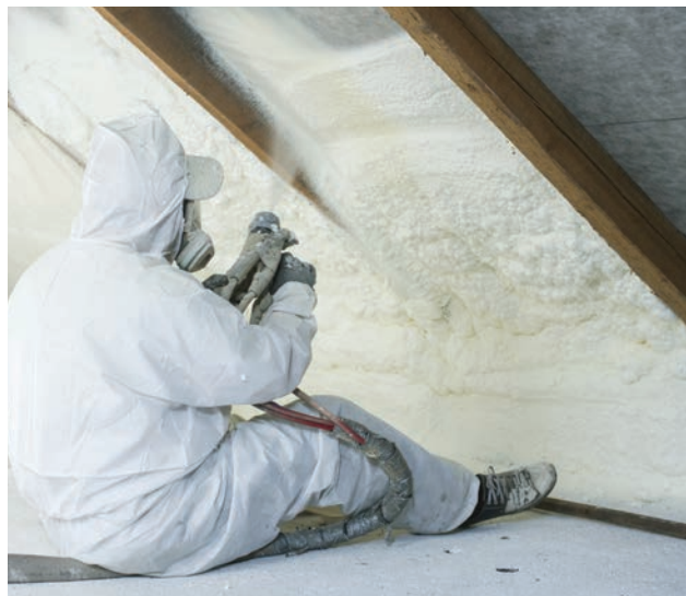
Spray foam installation in attic.
