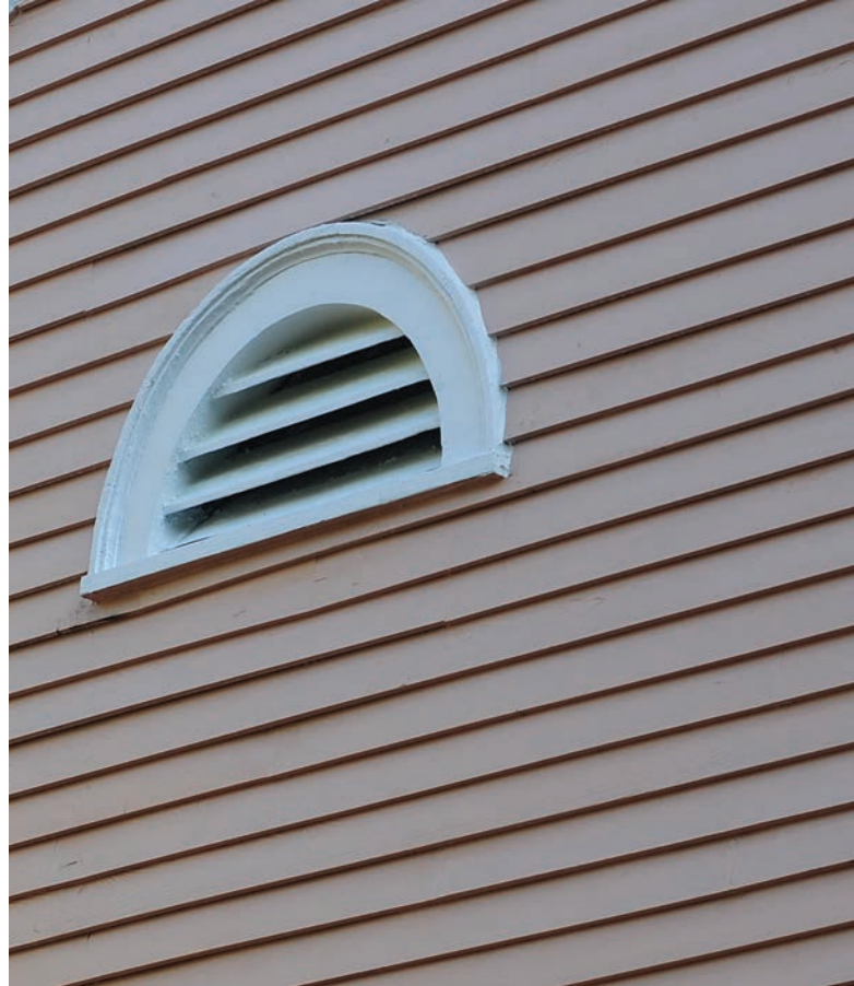
Attic eaves and venting.
