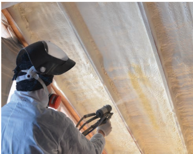
Spray foam installation.
