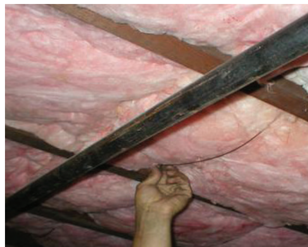
Fiberglass basement.
