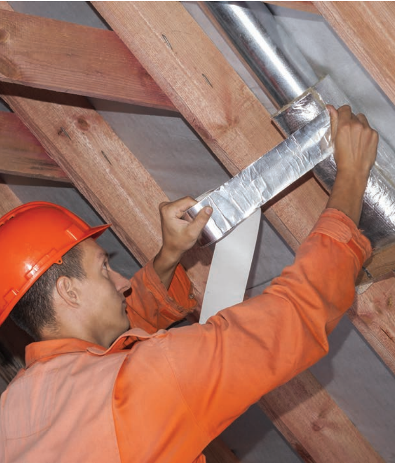
Sealing ducts.
