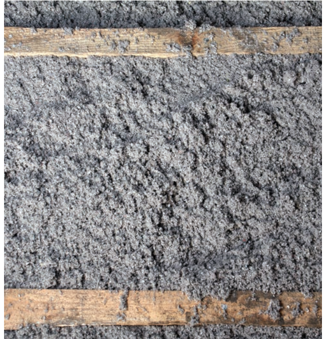
Cellulose insulation.
