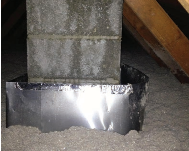
Flashed chimney with 3-inch spacing.
