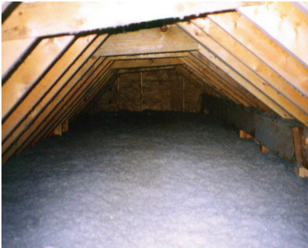
Loose-fill attic insulation evenly installed.
