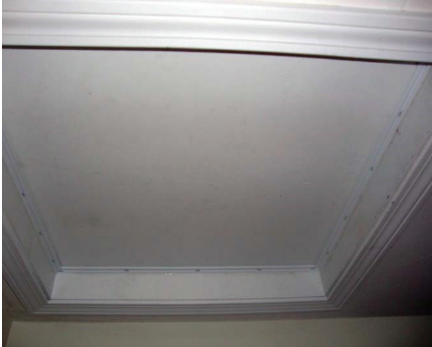
Attic hatch weatherstripped.
