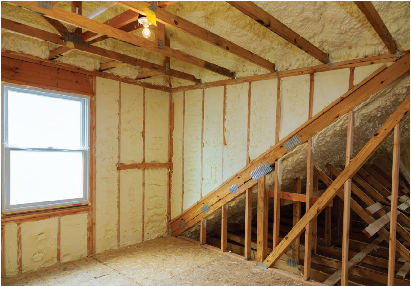
Spray foam installation.
