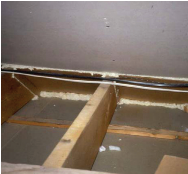
Knee wall attic air sealed along rafter line.
