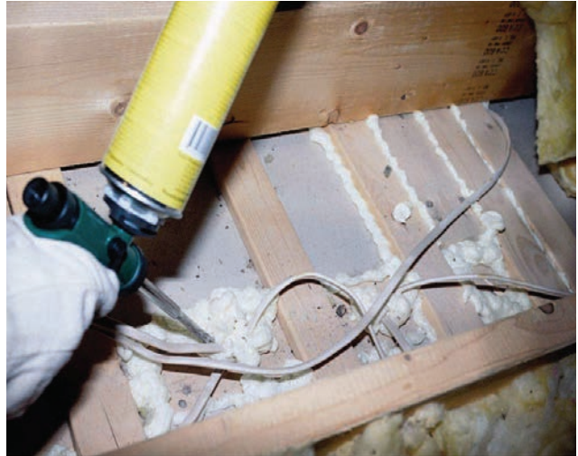
Top plates sealed with one-part foam.
