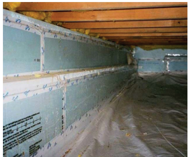
Crawlspace ground cover.
