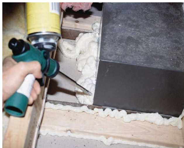
Bath fan sealed with one-part foam.
