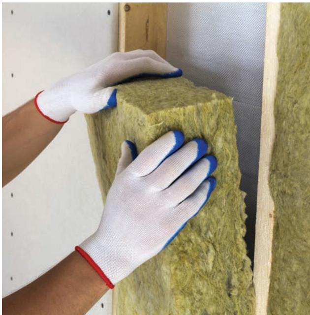
Insulate wall framing.
