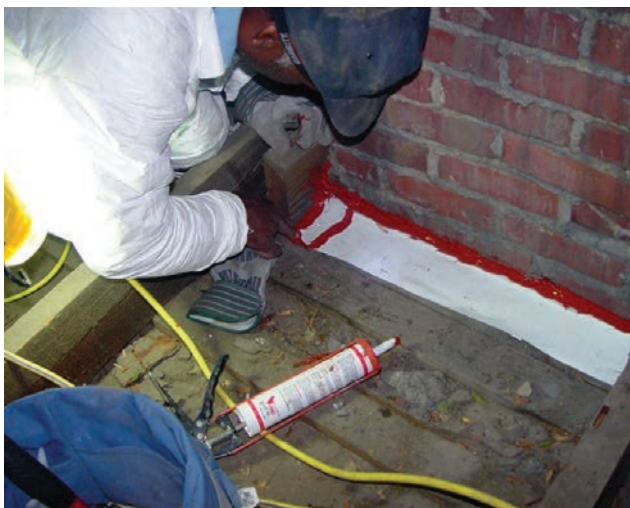
Chimney in attic sealed with high-temp caulk and metal flashing.
