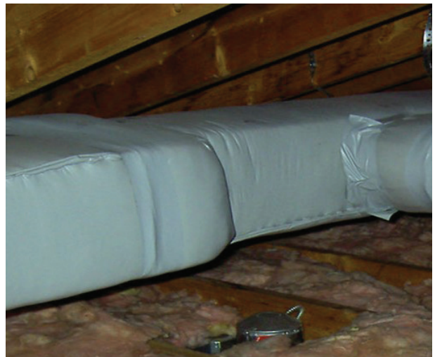
Sealed vapor retarder on attic ductwork.
