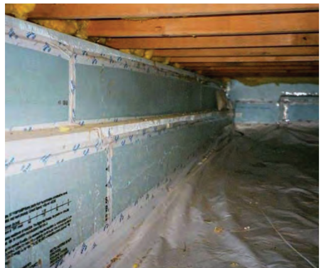
Crawlspace ground cover.
