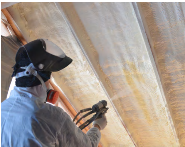
Spray foam installation.
