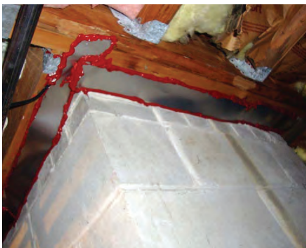
Chimney in basement sealed with sheet metal and high-temp caulk.
