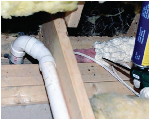
Plumbing wet wall sealed with fiberglass batt backer and one-part foam.
