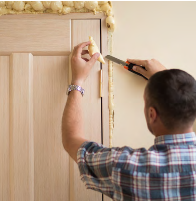
Clean up spray foam air sealing around doors.
