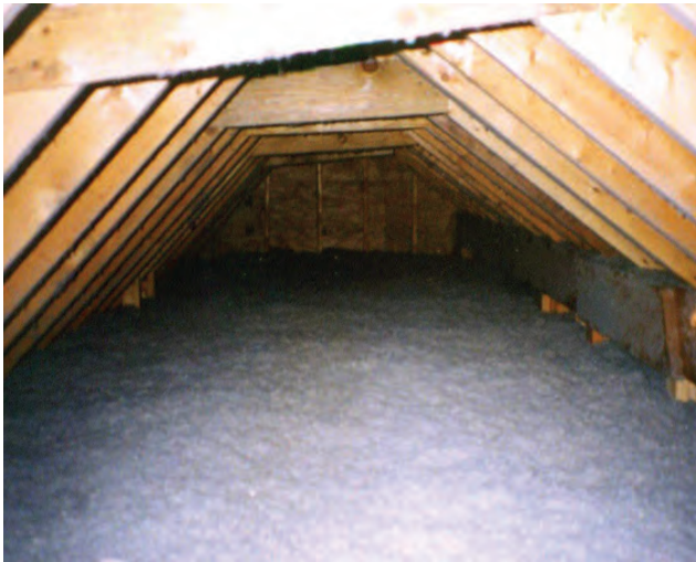
Loose-fill attic insulation evenly installed.
