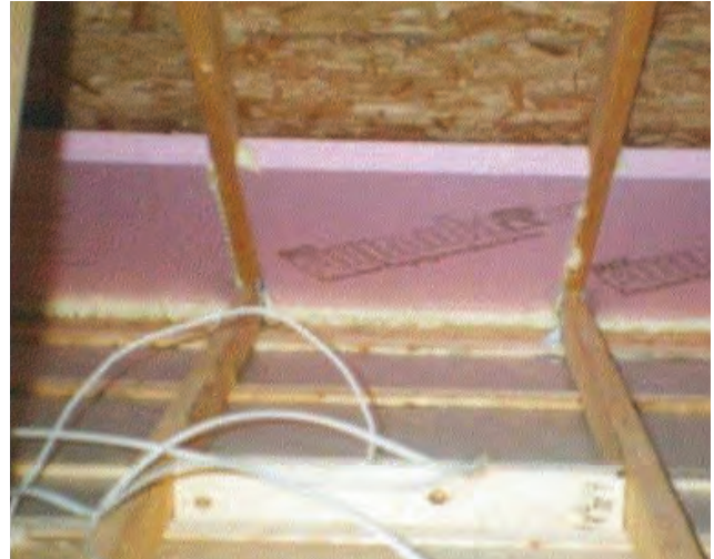
Insulation wind wash baffle.
