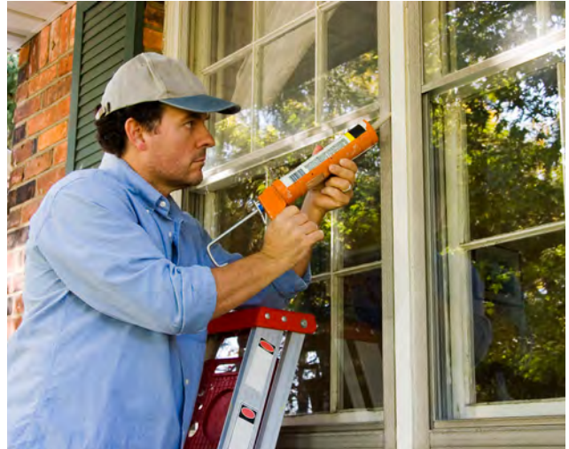
Applying caulk around window frame.
