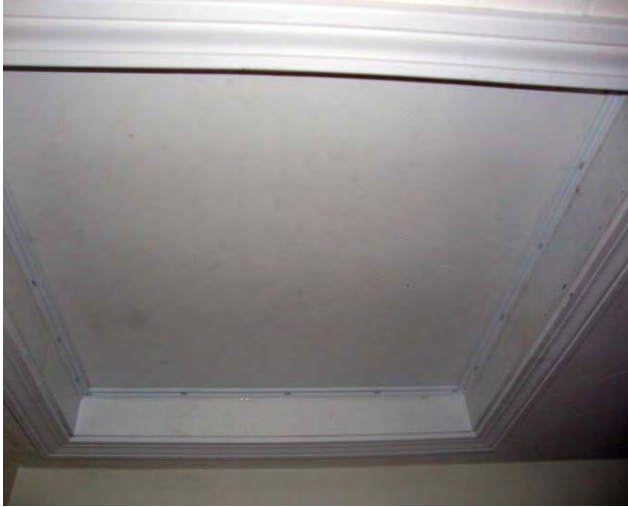
Attic hatch weatherstripped.
