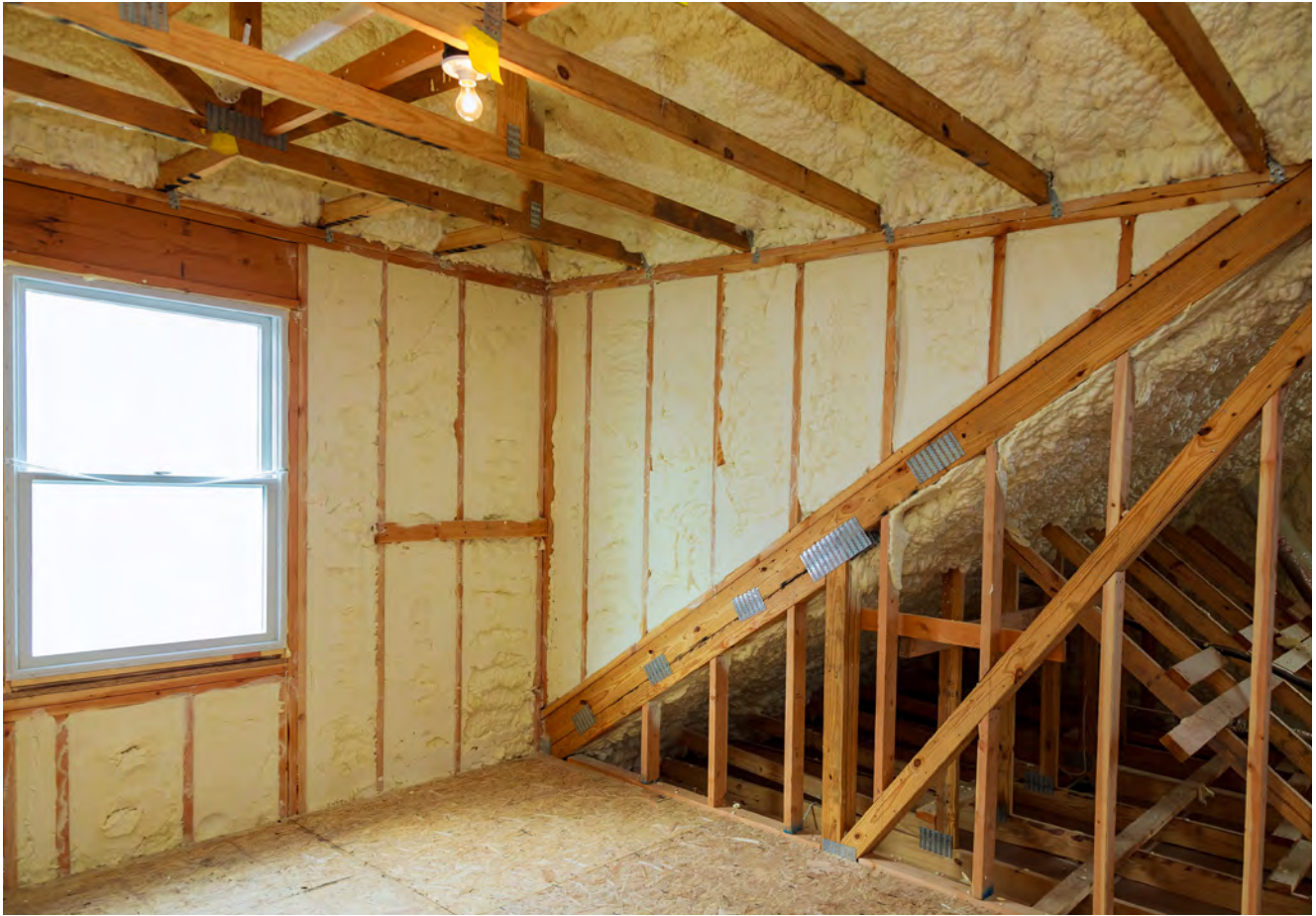
Spray foam installation.
