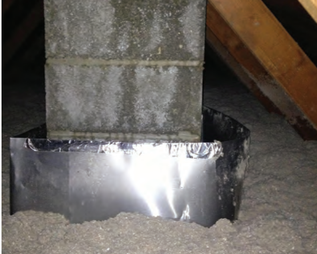
Flashed chimney with 3-inch spacing.
