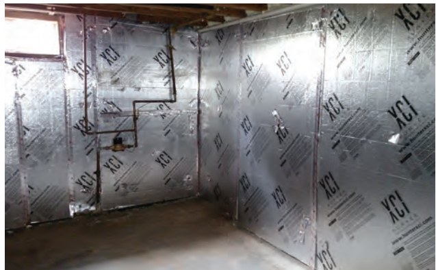
Basement and crawlspace insulation interior wall treatment.
