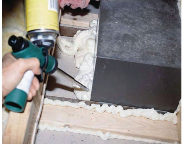
Bath fan sealed with one-part foam.
