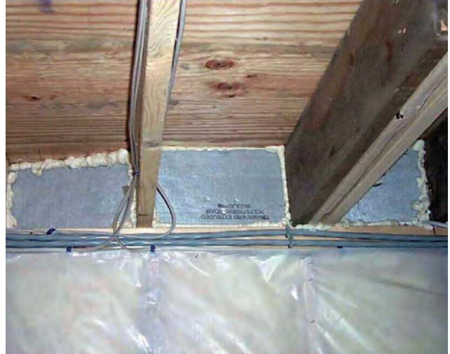
Rim joist sealed to sill.
