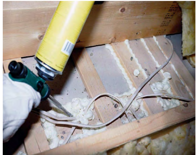
Top plates sealed with one-part foam.
