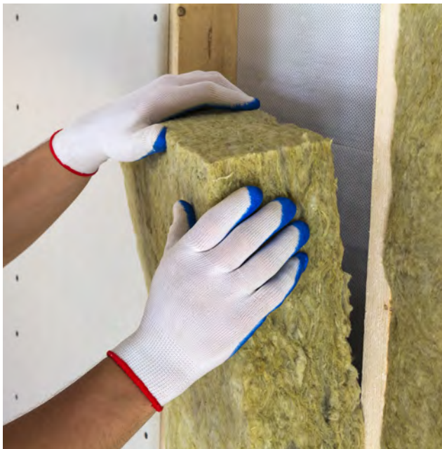
Insulate wall framing.
