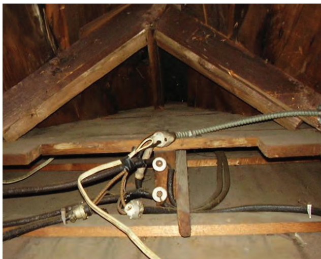
Knob and tube wiring.
