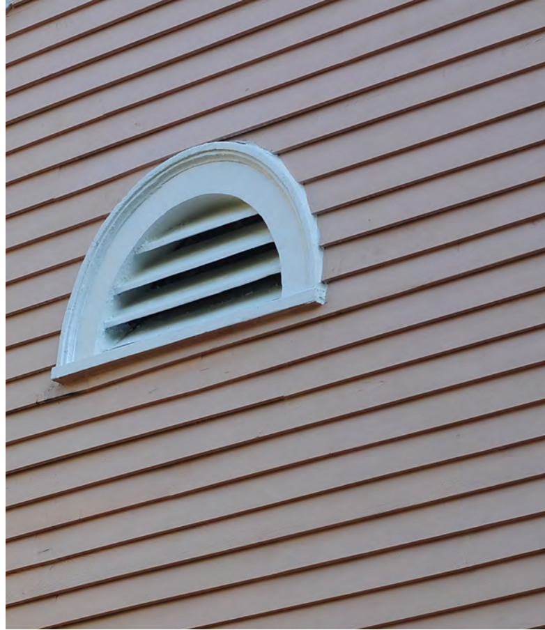
Attic eaves and venting.
