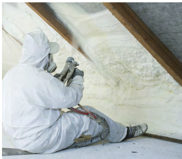
Spray foam installation in attic.
