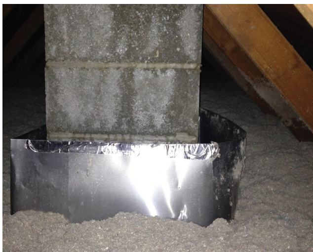
Flashed chimney with 3-inch spacing.
