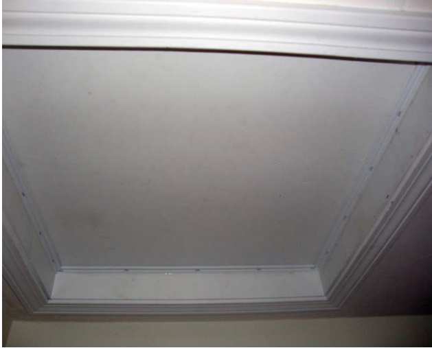
Attic hatch weatherstripped.
