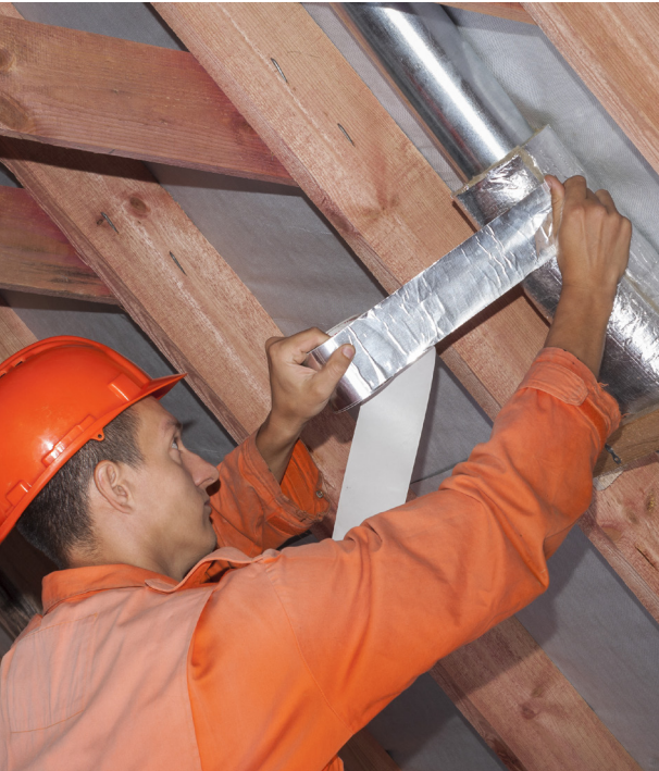
Sealing ducts.
