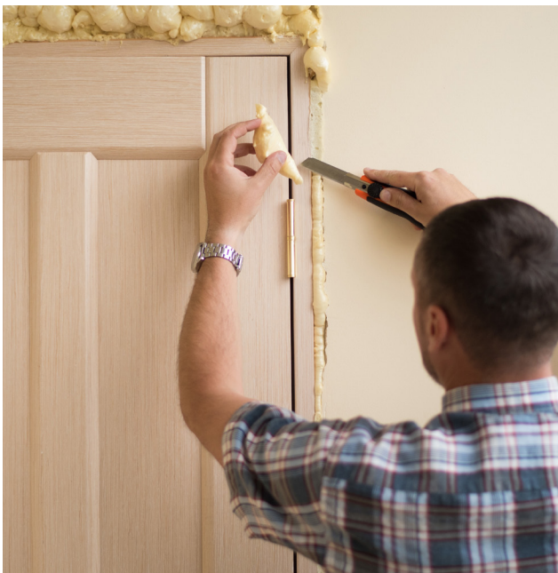
Clean up spray foam air sealing around doors.
