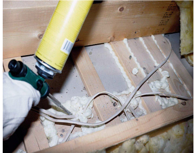
Top plates sealed with one-part foam.
