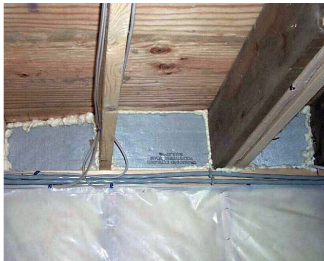
Rim joist sealed to sill (and insulated) with foam board and one-part foam.
