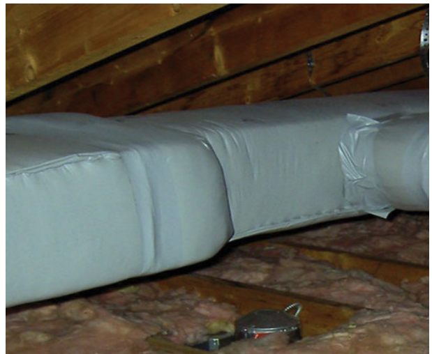
Sealed vapor retarder on attic ductwork.
