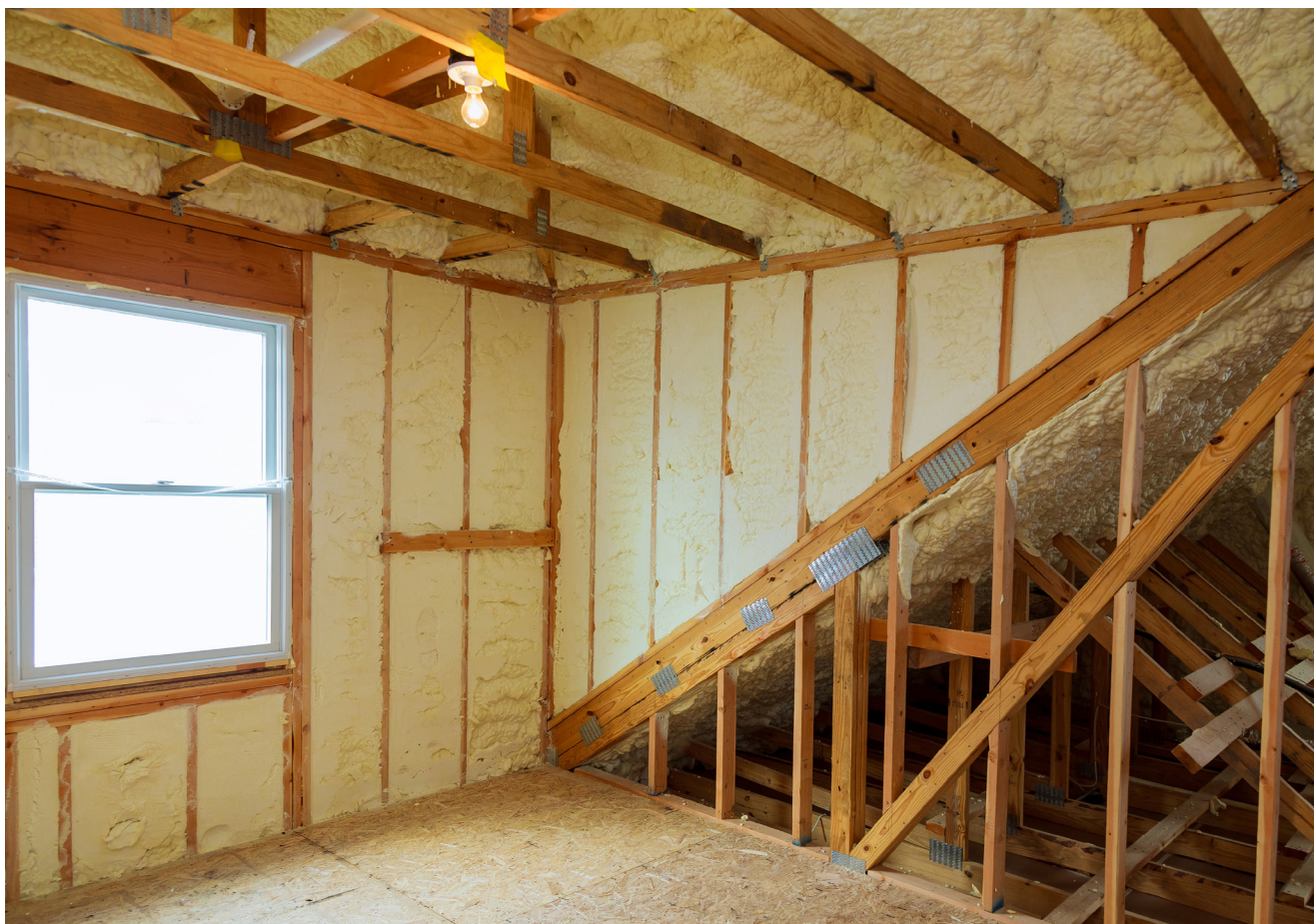
Spray foam installation.
