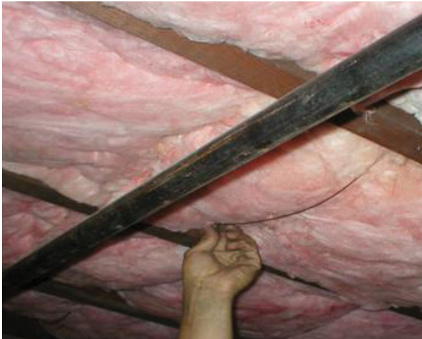
Fiberglass insulation in basement.
