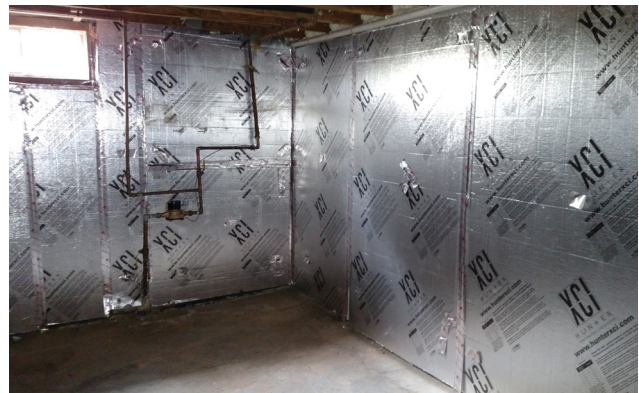
Basement and crawlspace insulation interior wall treatment.
