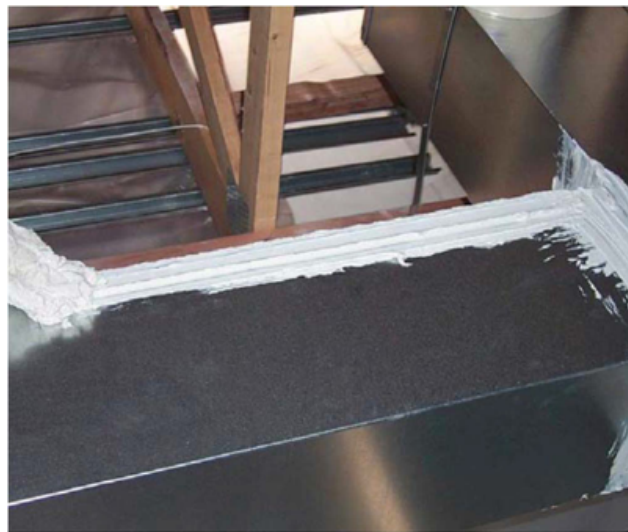
Metal ductwork sealed with mastic.
