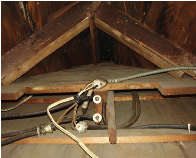
Knob and tube wiring.
