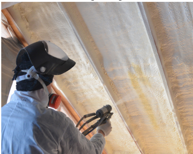
Spray foam installation.
