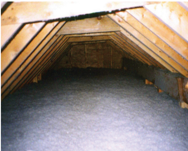
Loose-fill attic insulation evenly installed.
