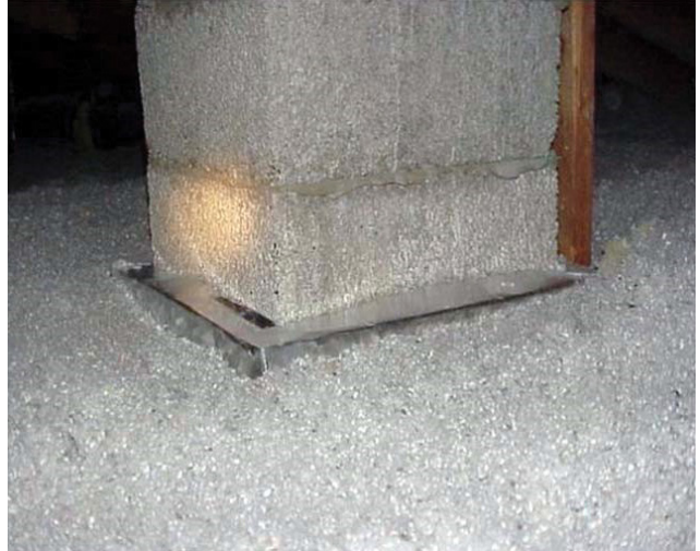
Attic insulation dammed away from chimney.
