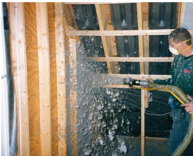
Roof line venting chute.
