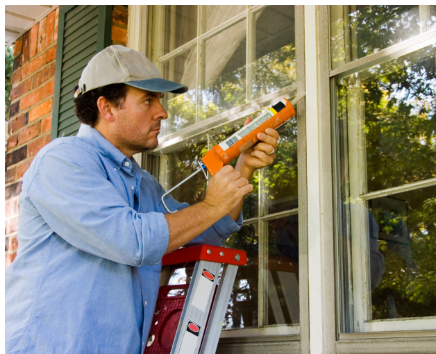
Applying caulk around window frame.
