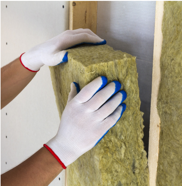
Insulate wall framing.
