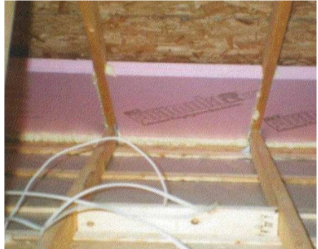
Insulation wind wash baffle.
