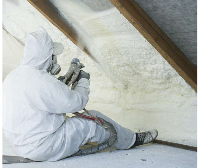
Spray foam installation in attic.
