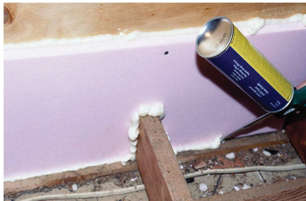
Knee wall transition sealed with XPS and one-part foam.
