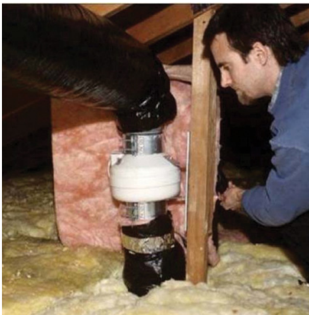
In-line exhaust fan ventilation.
