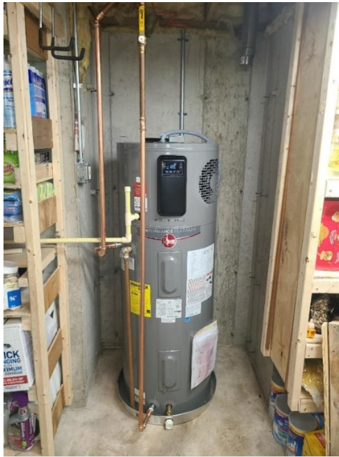
Figure 17. A KJM Plumbing HPWH Installation
